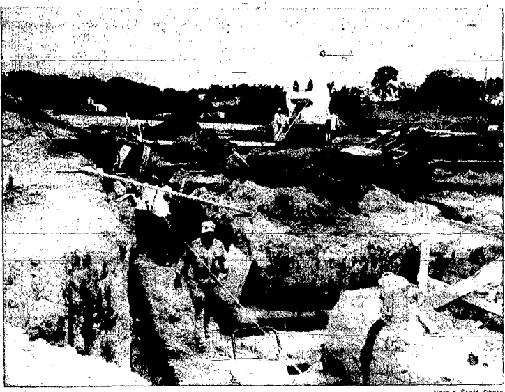
WORK ON WAYNE'S new elementary school was Fifth street. The view pictured above is looking well underway this week as workmen poured footings for the structure. The new building, which probably will be ready for use in the fall of 1960, is located on a 10-acre tract at the west end of Fifth street.
